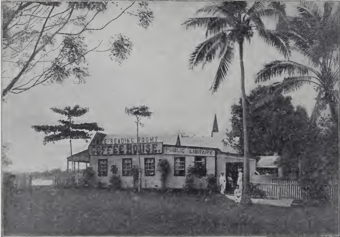
VIEW OF THE COFFEE HOUSE FROM THE MISSION COMPOUND.
